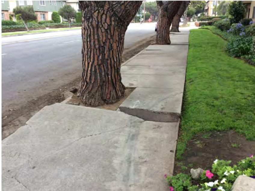
Example 4 – Existing Conditions
