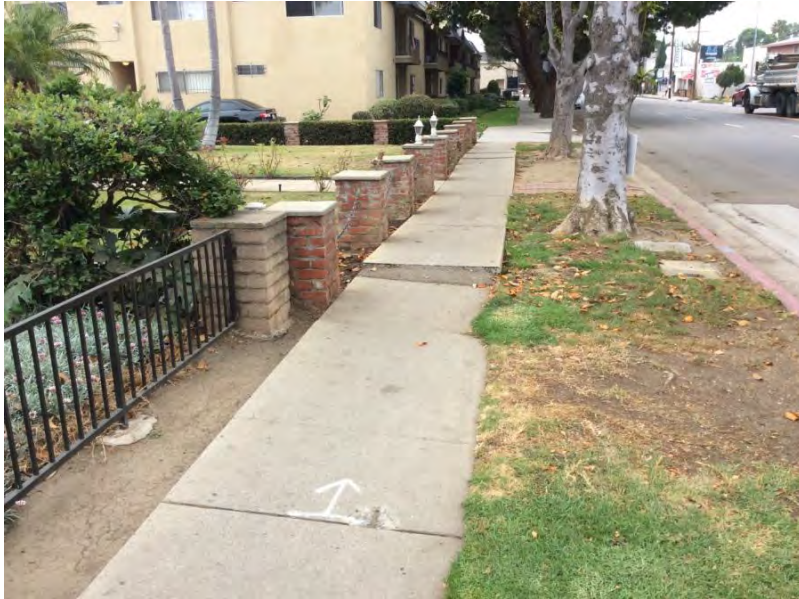
Example 3 – Existing Conditions
