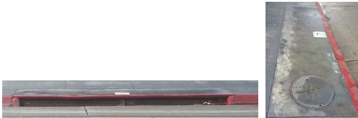
Example of a Typical Catch Basin
