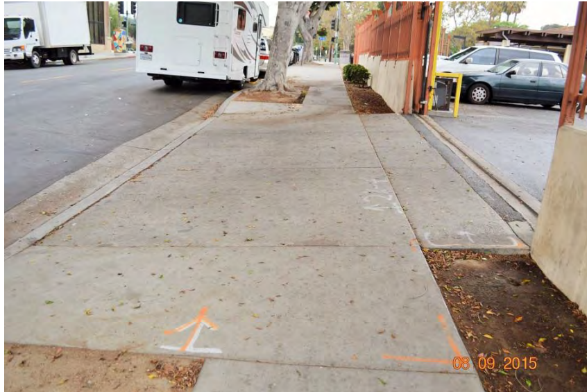
Example 5 – Existing Conditions
