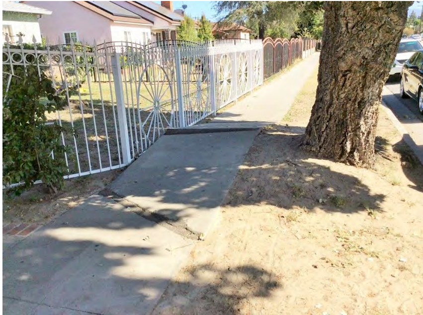
Example 1 – Existing Conditions
