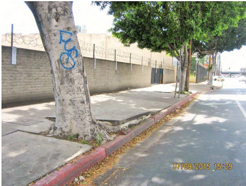
Example 6 – Existing Conditions
