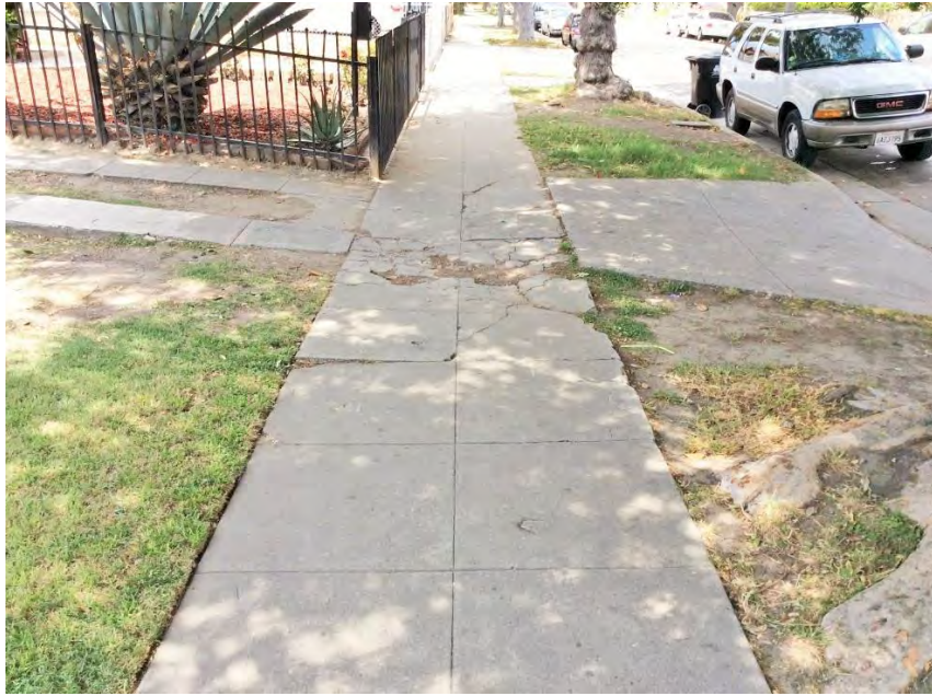
Example 2 – Existing Conditions
